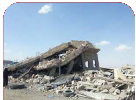
A part of the destruction caused to the targeted house
