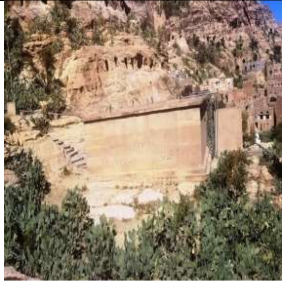
The main water storage tank in Shibam City, Shibam Kawkaban District, Al-Mahwit Governorate.
