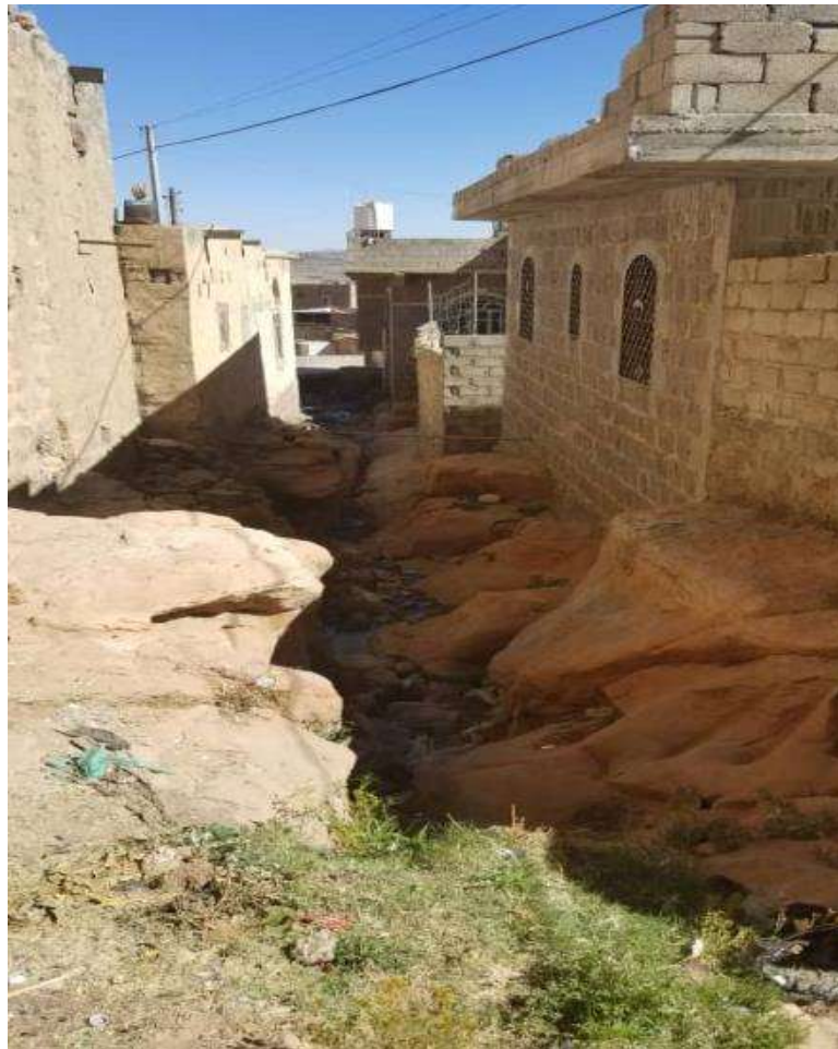
Photo: Sewage discharge between houses
