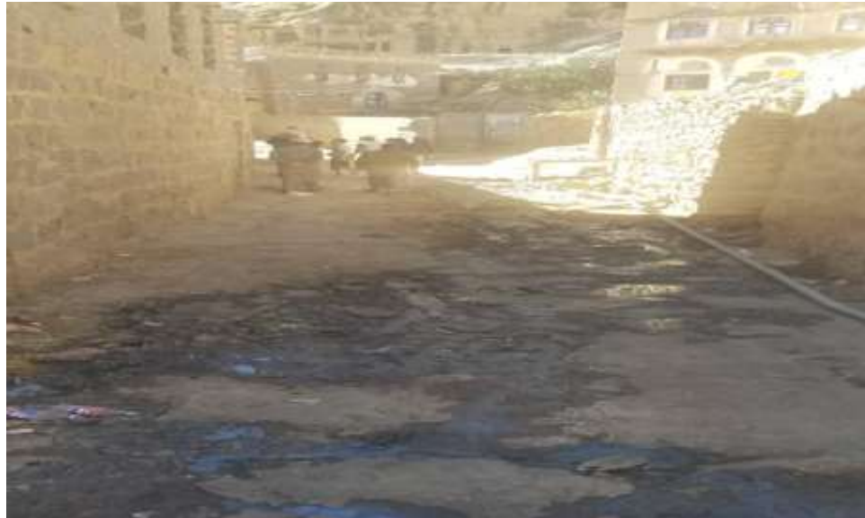
Photo: Sewer drainage between houses in the community
