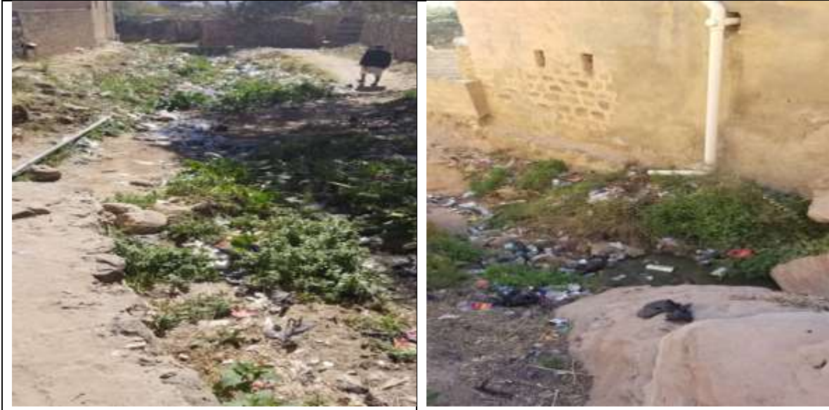
Open drainage observed next to houses in Shibam City.
