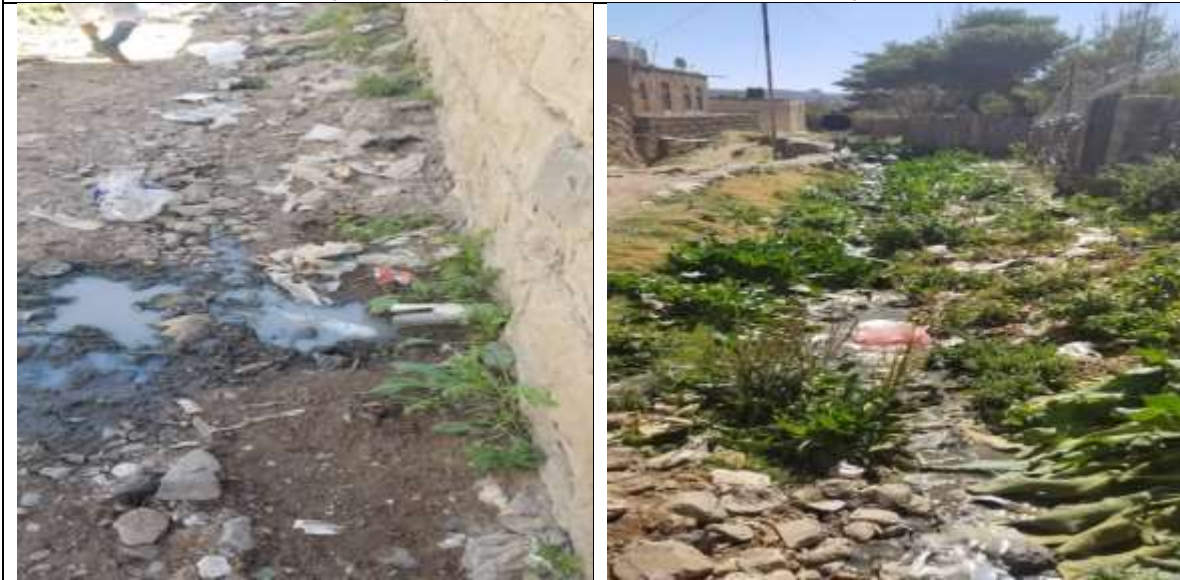
Sewage discharge between houses as well as rain/water streams in Shibam City.
