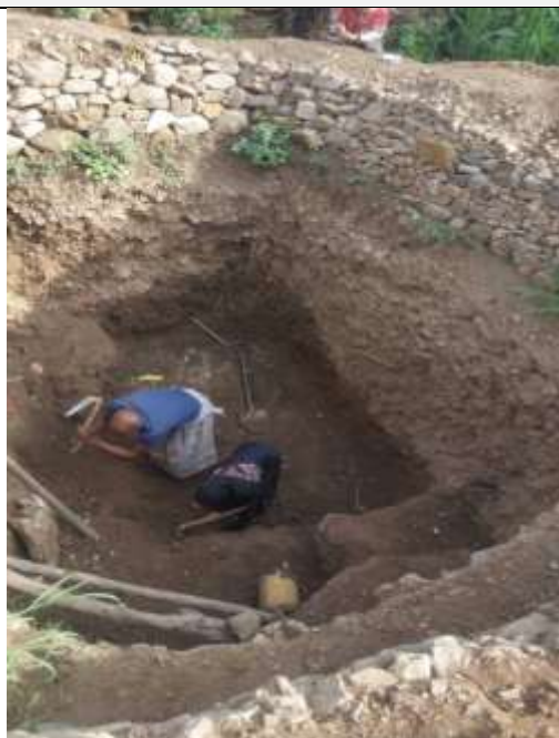
Photo (4) Pit latrines digging by HHs – RRT photo
